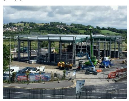
b. Once this was completed, a new exterior – of walls, cladding and windows – was constructed. The building was then completely re-roofed.
